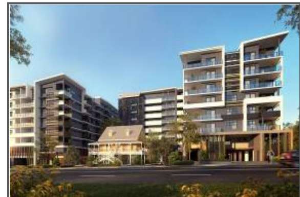
Topaz Residences, including the restoration of the heritage-listed Abbotsford House is the latest addition to Devine Constructions' workbook
